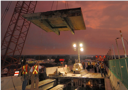
Rehabilitation of the Laviolette Bridge. The work involved replacing over 325 m of slabs and 22 slabs of 30 m of prestressed concrete girders and slabs on the rest of the bridge section with steel girders and new slabs.
